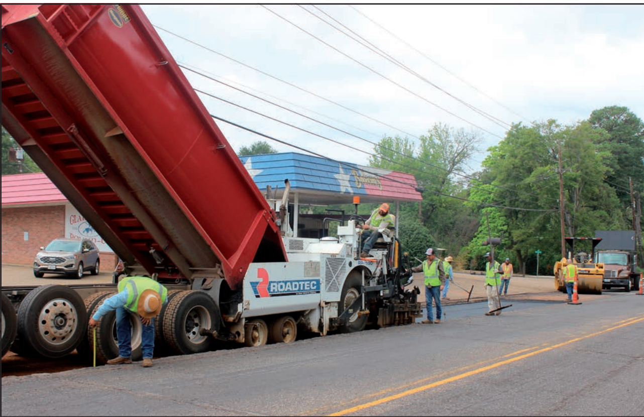
A road construction crew lays asphalt on Hwy. 80 east of W. Pacific Ave. Monday morning. Projects on the highway are spearheaded by Texas Department of Transportation. Photo by James Draper
