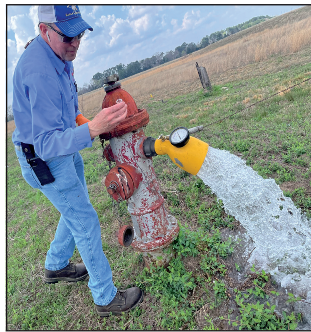
Water Plant Operator Nate Palmer takes a water sample Monday afternoon while flushing a hydrant on Hwy. 271 south of town.
