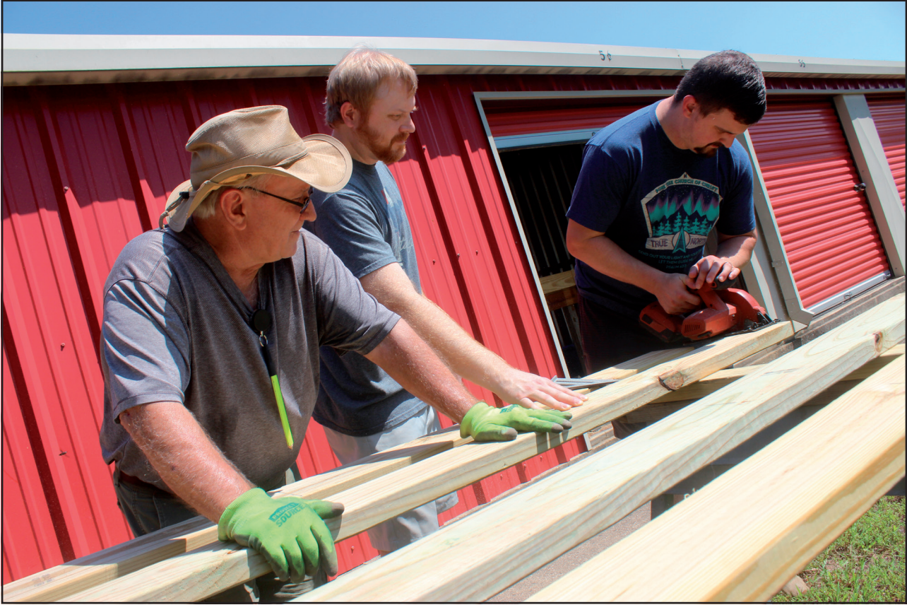
Gladewater Rotarians (from left) Leon Word, Sam Cloud and Nathan Burkhalter assemble ramp modules Sept. 11, getting ready for this weekend’s local build in partnership with Texas Ramp Project.
