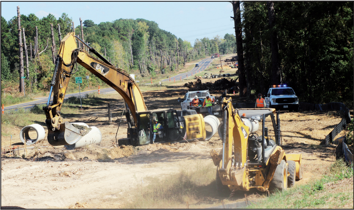
Construction crews work along George Richey Road (FM 2275) in White Oak, one step at a time to widen the route to four lanes plus a turn lane between White Oak Road and Pine Tree Road, ultimately to SH 300.
