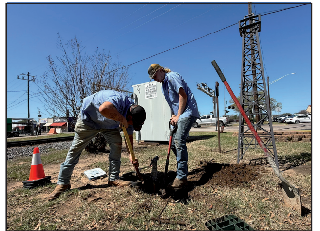
Gladewater Public Works employees Sam Loy and Jacob Glass check a copper and lead service line downtown March 19. All services in town will be checked as part of a regular report to the state.
