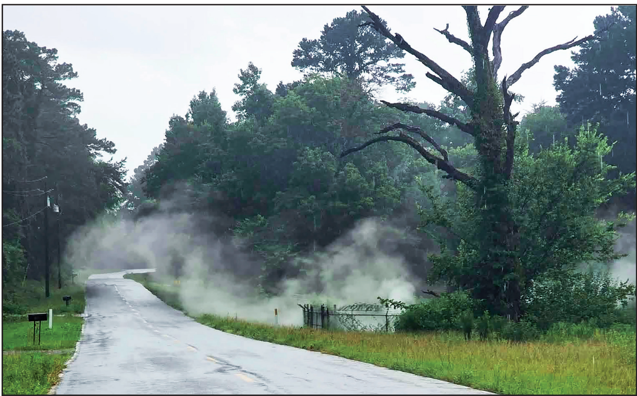
Moisture-heavy natural gas wreathes the roadway on Sheppard Lane Sunday afternoon after a falling tree ruptured a line serving the area. The weather prevented the gas from escaping into the atmosphere, Gladewater Fire Chief Tim Basham said, making the situation all the more dangerous. Residents in two nearby homes were evacuated while first responders and utility crew members worked about four hours to clear the scene.
