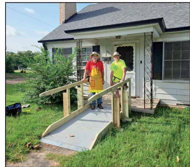
Gladewater Rotary Club members and other volunteers recently completed accessibility ramps for residents in need in both Gladewater and Liberty City. Courtesy photos from Gladewater Rotary
