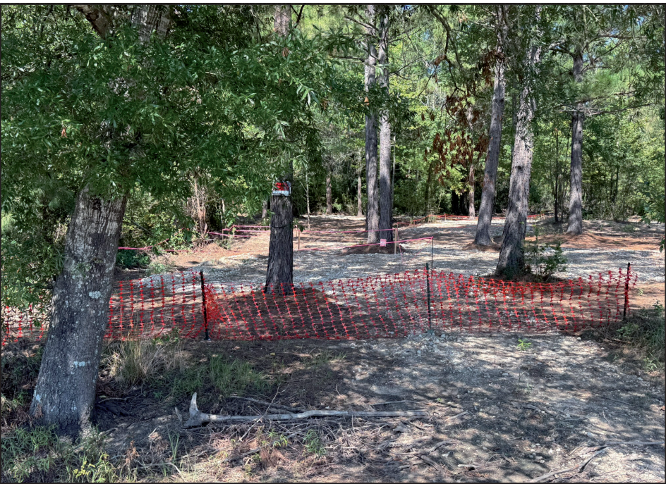
Work on the planned Dine and Pines Food Truck Park is paused after initial clearing on the corner of South Main Street and Loop 485. The developers applying for a Specific Use Permit, with a hearing scheduled at the Planning & Zoning Commission Thursday followed by council consideration Aug. 20. If approved, the Staerker Brothers LLC has already been green-lit for reimbursement of up to $30,000 through Gladewater Economic Development Corporation's Grow Gladewater Grant program.
